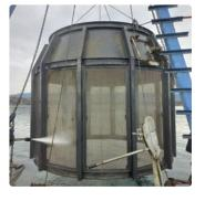
An entire year has passed since cleaning work was undertaken at the Prieuré plant and a new lining was added to the screen filter. The results have been very positive: with mussels no longer present, the screen filter can now be cleaned very easily just by rinsing it out.
